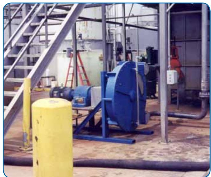
Abaque™ Series Peristaltic (Hose) Pumps feature a method of operation that is perfect for handling the of viscous, abrasive or particulate-laden fluids that are a staple of the mining industry.
