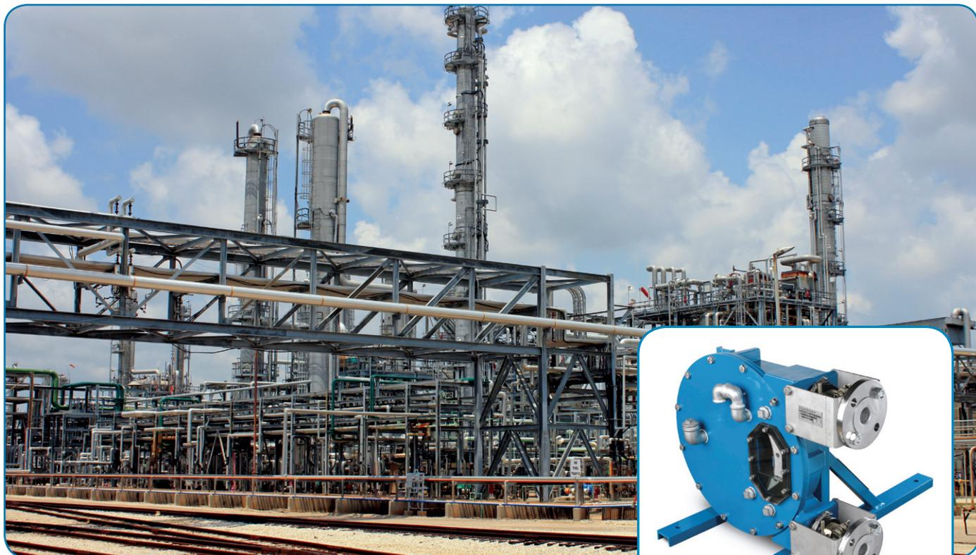
The sheer volume of chemicals that need to be produced to satisfy global demand in many industries requires the use of reliable, efficient and safe pumping technology, such as that offered by Abaque™ Peristaltic (Hose) Pumps (inset).
